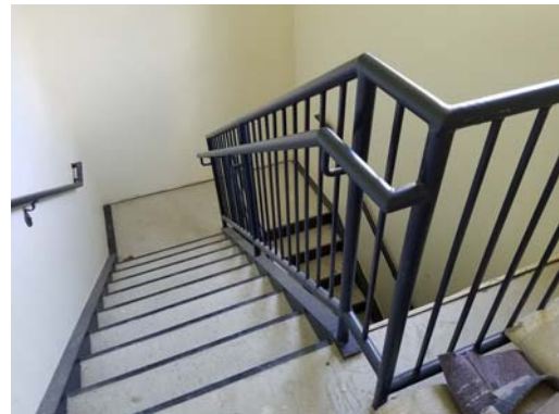
School to unfinished space stairway
